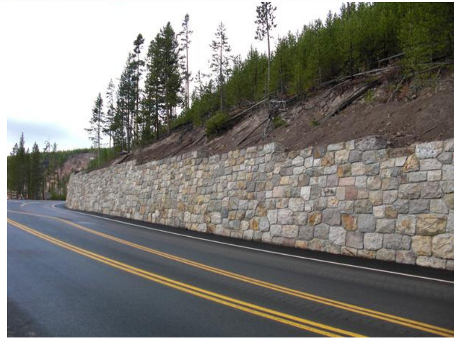
Cut stone masonry wall in Yellowstone Nat'l Park
